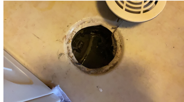
Sluk mangler klemring
