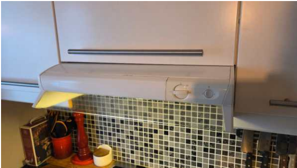
Ventilator over kokeplate.
